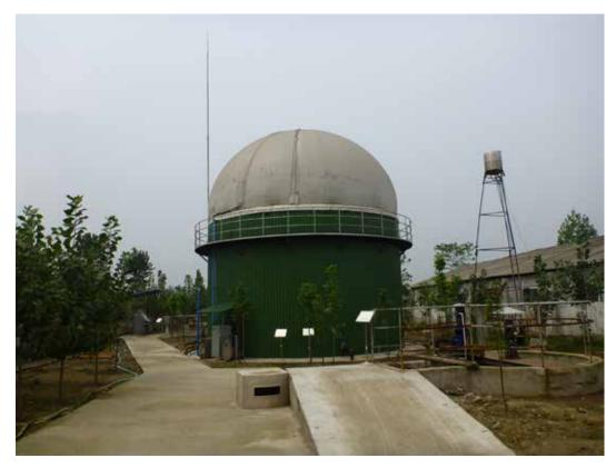
400 cublic meter biogas digester with flexible storage membrane on top.
