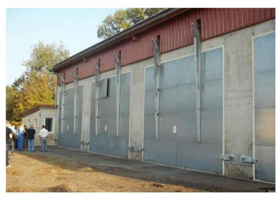
Garage digester showing individual 'garage' chamber doors. These doors are hinged at the top.
