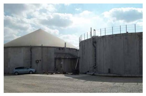
Biogas digester with flexible membrane storage vessel on the left.
