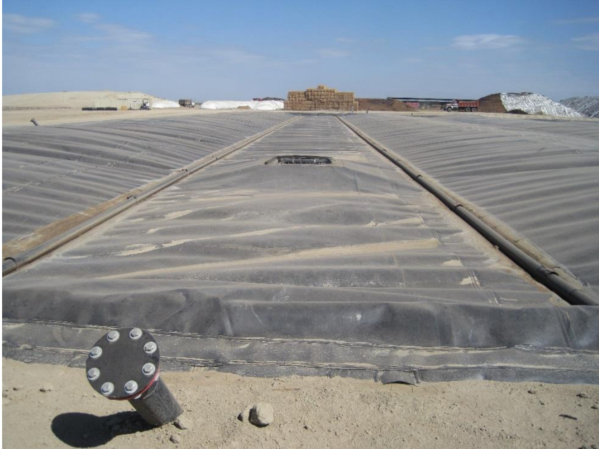
Figure 3: ABEC #3 Digester Cover Installation
