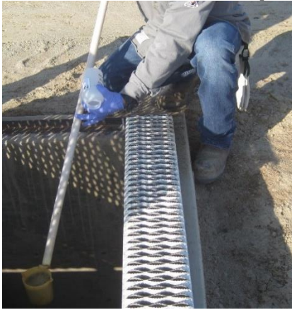
Figure 7: ABEC #3 Effluent Overflow Sump and Sampling Point
