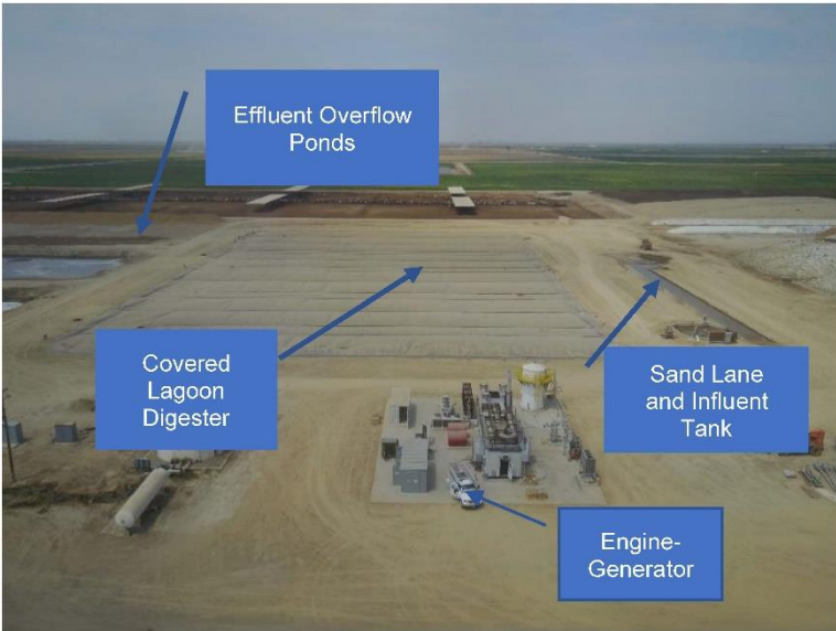
Figure 4: ABEC #3 Overview of Digester System
