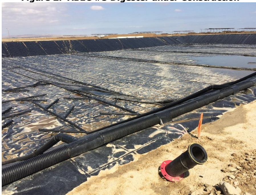
Figure 2: ABEC #3 Digester under Construction
